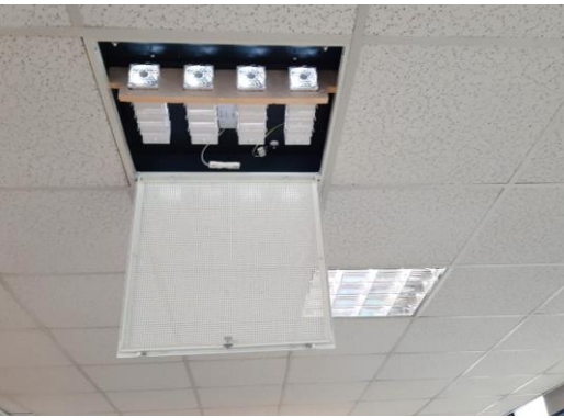
SANIXBOX INSERTED IN THE FALSE CEILING (60x60cm)
