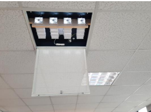
SANIXBOX INSERTED IN THE FALSE CEILING (60x60cm)
