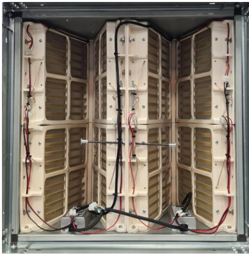
Filter holder counter frame with locking springs for corrugated G4 prefilter
